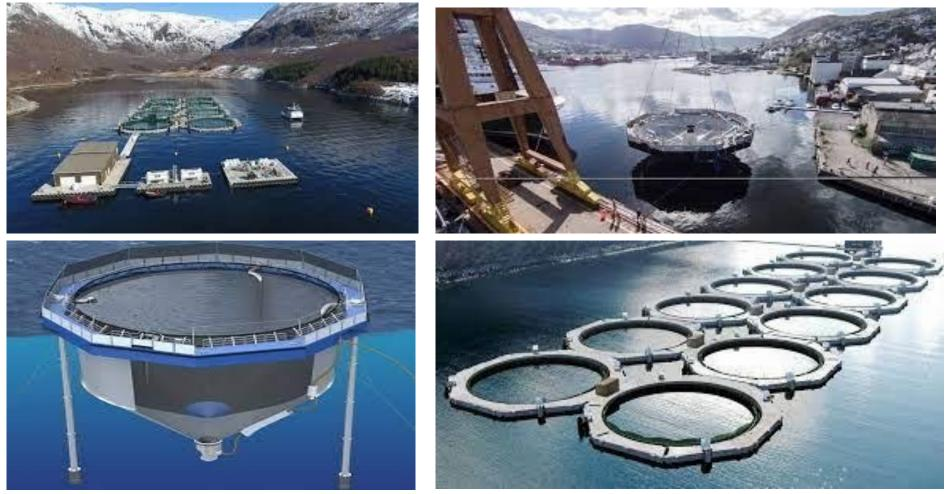
Illustration; Floating bags with dimension from 6 000m<sup>3</sup> to 30 000 m<sup>3</sup>. Pumping cost is 1 kwh per 1 kg fish produced<sub>29</sub> the same cost in Tanks on land is > 300- 600%.
